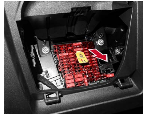
Cut-out connection in the passenger compartment, on the fuse carrier in the dash panel
